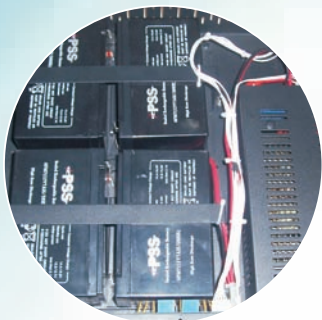
Batteries Installed
